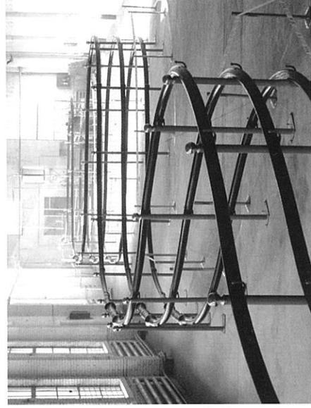
FIGURE 12.56: Pulling Southwire's triaxial cable into a cable duct at AEP's Bixby substation near Columbus, Ohio. (Courtesy Southwire Corporation.)
